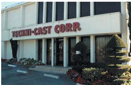
Techni-Cast Corp., a foundry based in South Gate, Calif., has met some of the nation’s toughest emissions requirements in a creative combined-heat-and-power project, with emissions solutions provided by MIRATECH.
