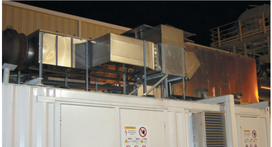
Techni-Cast emissions solutions include both a MIRATECH Selective Catalytic Reduction (SCR) system for NOx compliance, and a Non-Selective Catalytic Reduction System, the MIRATECH Oxidation Catalyst, for CO, HC, VOCs and HAPs compliance.
