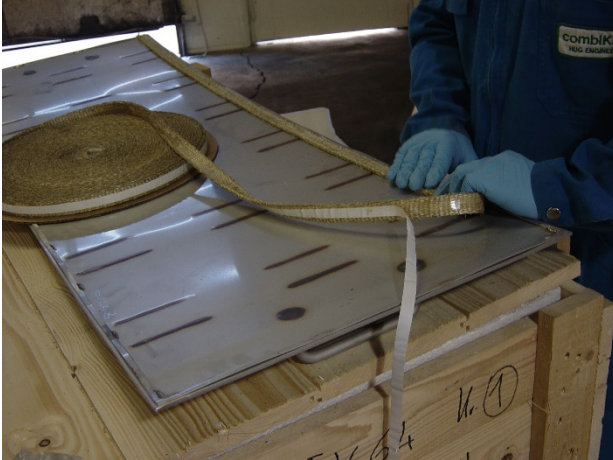
Figure 36: Installing Gasket Material
