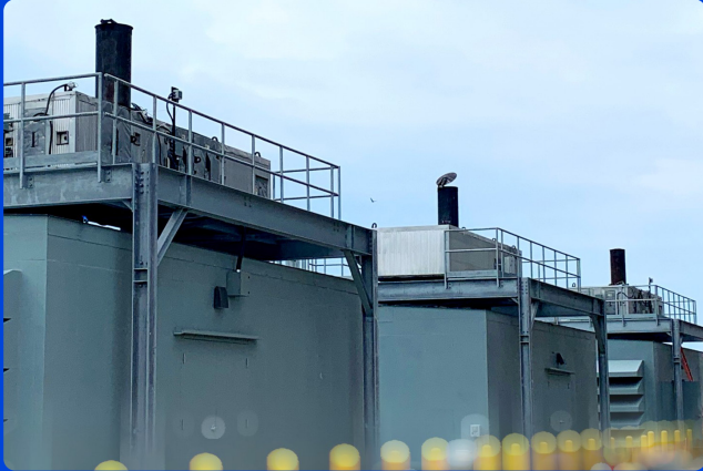
DATA CENTER INSTALLATION
